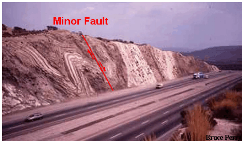
Picture of the Palmdale Road cut, with illustration of one of the many minor faults.
